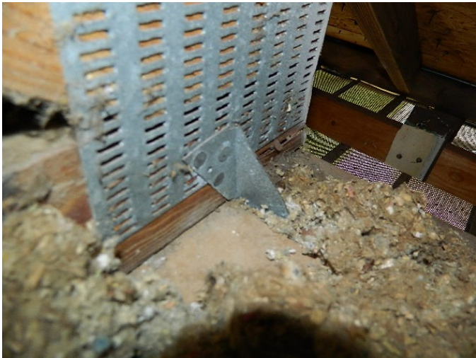
Roof to wall connector w 3 plus nails
