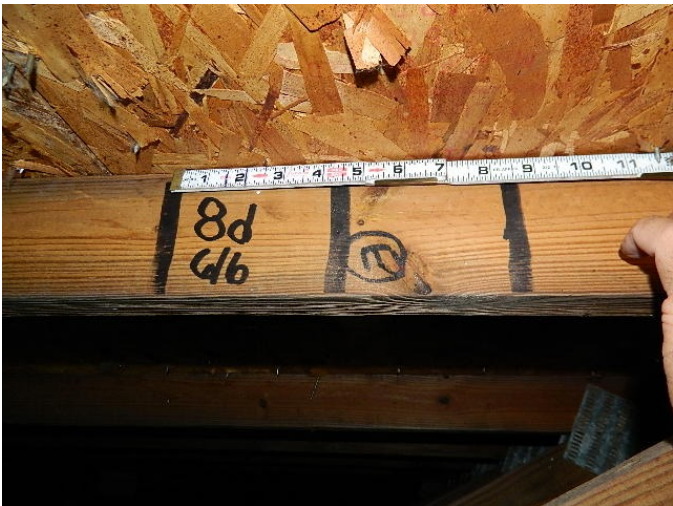
Roof deck attachment 8d nail 6/6
