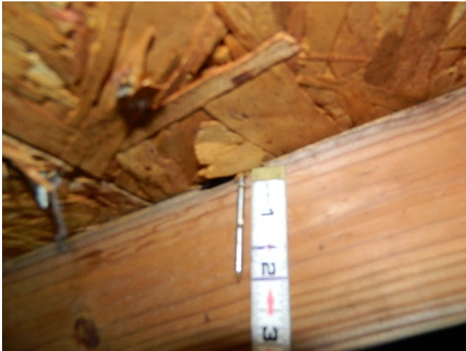
Roof deck attachment 8d nail
