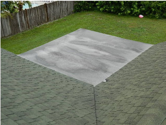
Roof covering, fiberglass shingle & bitumen roof
