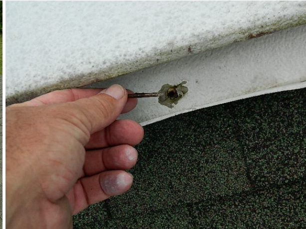
Fiberglass shingle and bitumen roof media along with loose ridge vent
