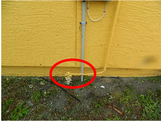
Electrical panel main ground and possible overheated main/oxidized
