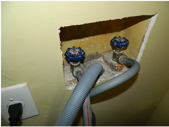
Washing machine and utility sink water shut off valves
