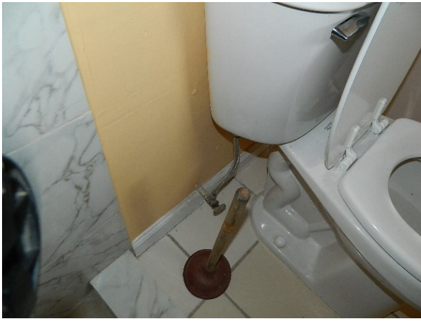
Master bathroom toilet and vanity water supply line shut offs
