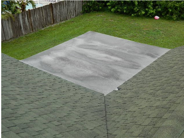
Fiberglass shingle and bitumen roof media along with loose ridge vent
