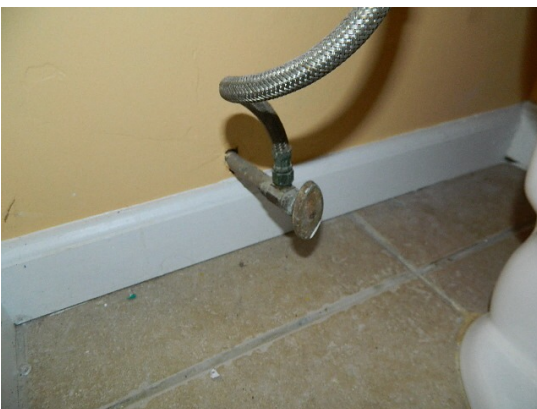
Hall bathroom toilet and vanity water supply shut offs
