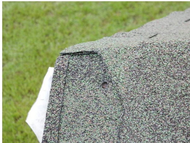
Missing ridge cap and shingle wear due to tree branches
