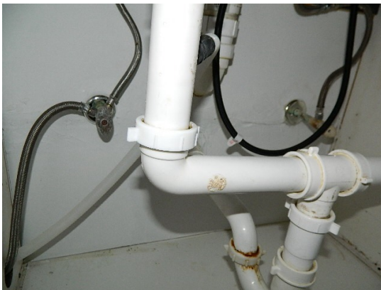
Kitchen sink water supply shut off valves
